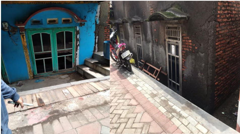
Figure 4. Physical adaptation of infrastructure buildings due to tidal floods
