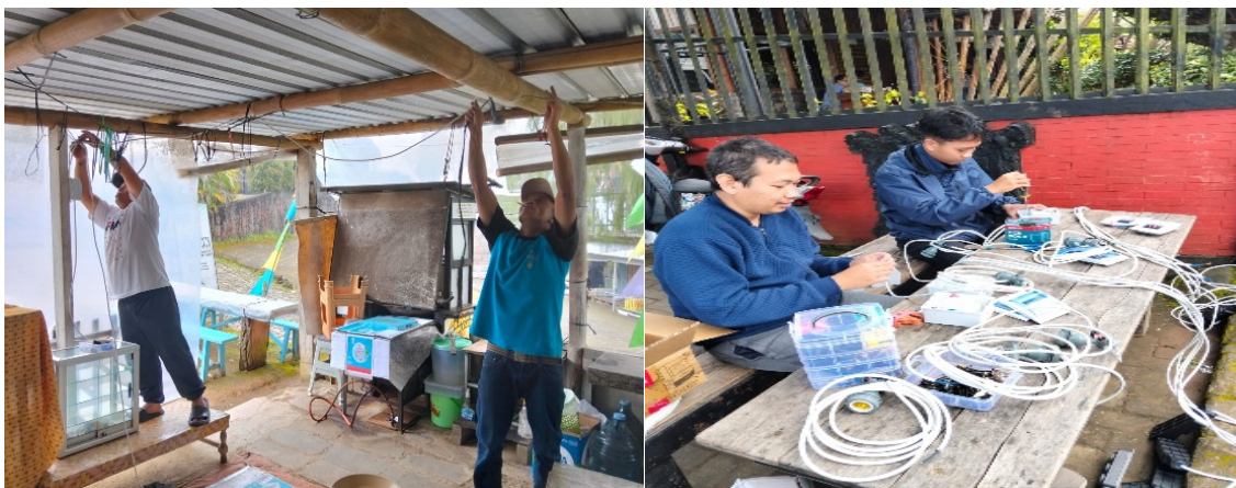
Figure 4. Installation of installations at Posong Nature Tourism
