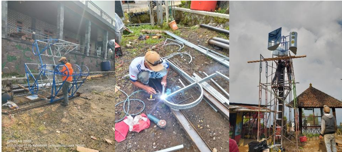
Figure 5. Welding and assembly activities of wind turbines on the tower
