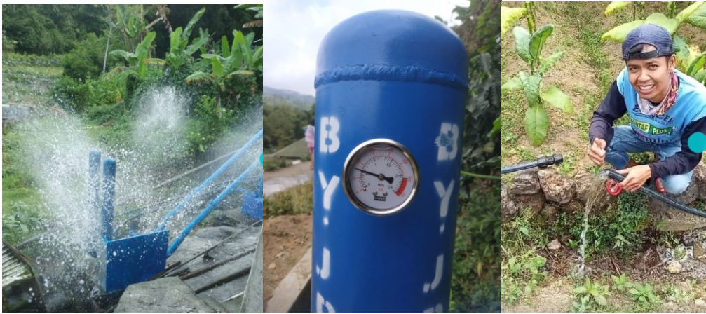
Figure 8. Smart Hydra Twin Flow system combining two hydraulic ram pumps with a stabilizer tube to lift water through a vertical elevation of up to 190 meters in Tlahap Village
