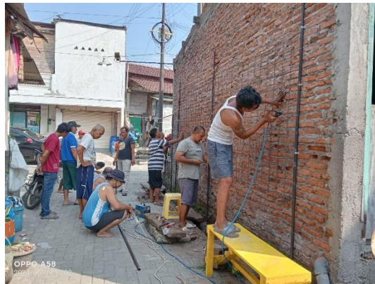
Fig. 5. Creation of wire mesh for the vertical garden
