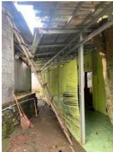
Figure 1. Photo Building Condition
