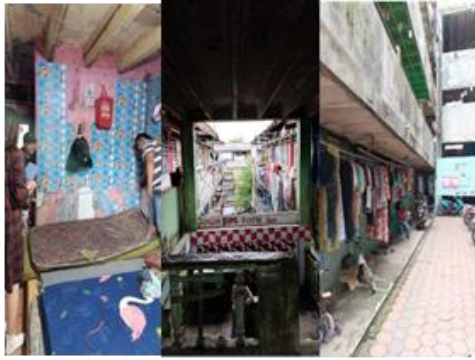
Figure 1. Existing Conditions of the 24 Ilir Housing Complex in Palembang City
