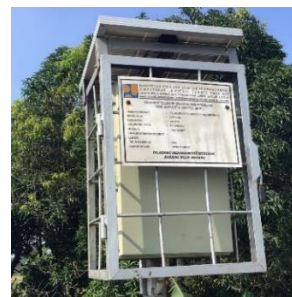
(2) Telemetry Open Standpipe Piezometer 7
