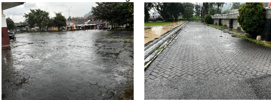
Picture 9. Small Sections of Alun-Alun Bung Karno Using Paving Blocks
