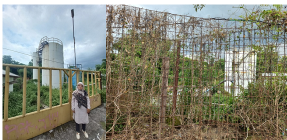
Figure 4. IPAL (Waste Water Treatment Plant) which is no longer operational
