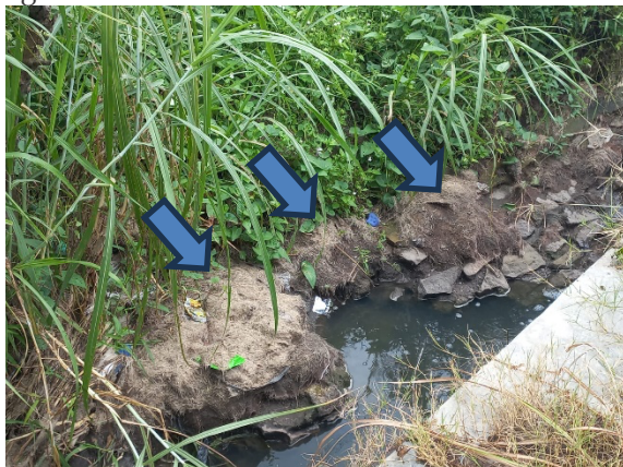
Figure 7. Pati Onggok Solid Waste which Interferes with Irrigation (shown by arrow)
