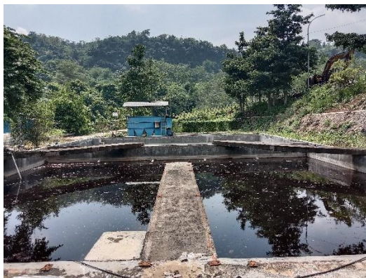
Figure 1. Jatibarang Landfill Leachate Pond
