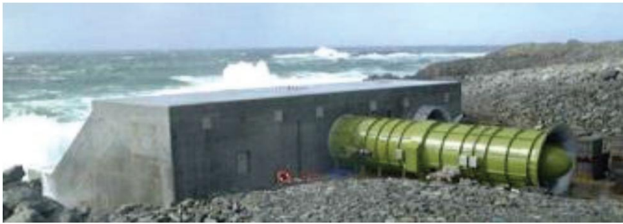
Figure 4. Prototype of LIMPET Constructed In 2000 on the West Coast Of The Scottish Island Of Islay [51]
