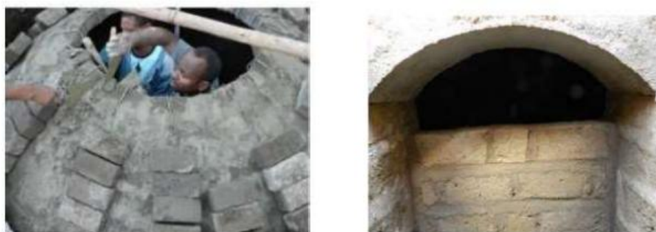
Figure 6. SINIDU 2008 dome construction (left), solid baffle introduced (right)
