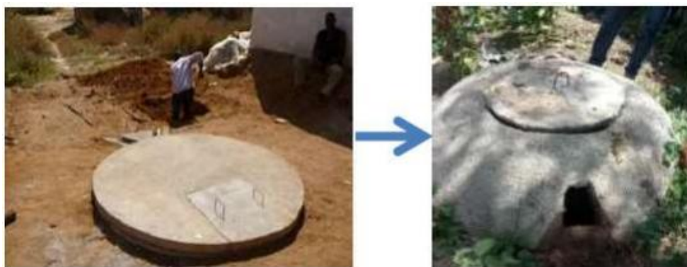
Figure 8. Before modification (left) and after modification (right)
