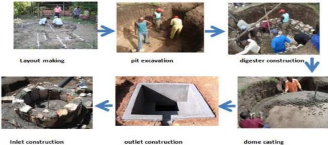
Figure 4. Major steps during biogas digester construction [4]
