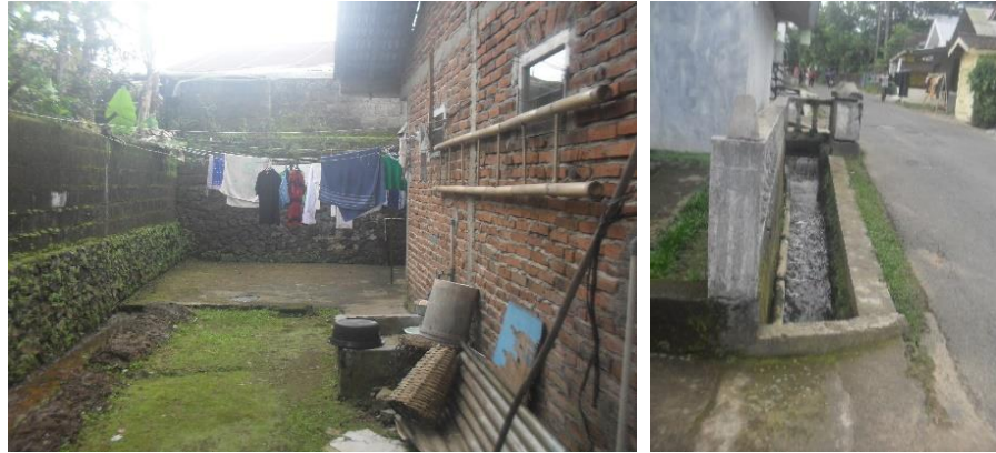
FIGURE 2. Clean Water Distribution System for Consumption and Clean Water Flowing, in the Back, and also Dirty Water Drain in Front of the House
