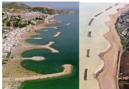
FIGURE 3. Sedimentation behind coastal protection structure [1]
