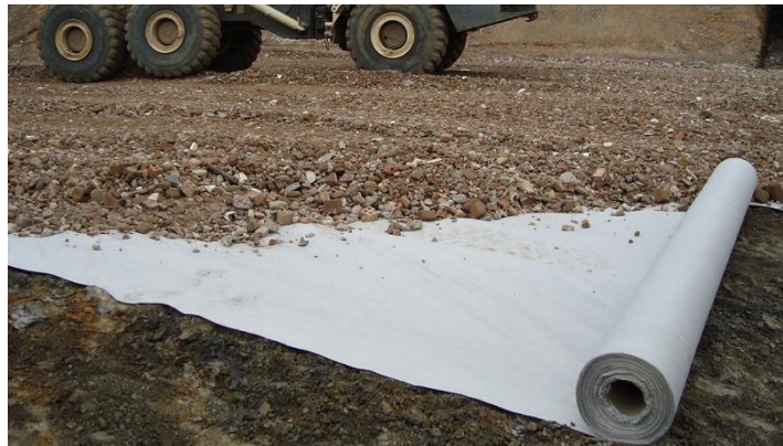
FIGURE 1. Non-woven geotextile (Source : Polyfabrics.com.au)
