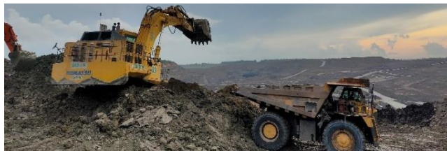
FIGURE 2. Heavy equipment loading process
