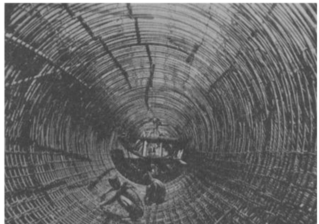
Figure 3. Laborers working on the construction of the Malahayu Reservoir. (Source: De locomotief, December 2, 1937)
