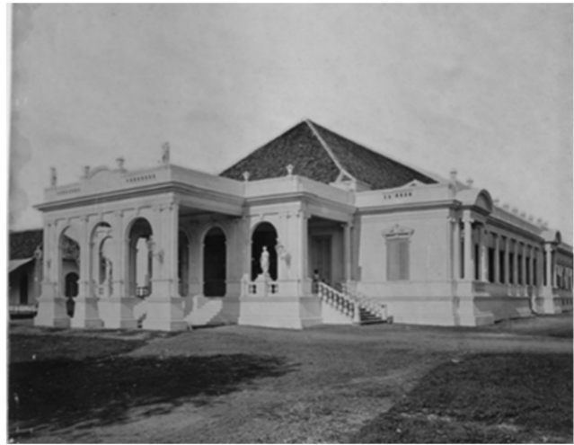
Figure 1. Kiritsu Gehitzzyoo Building, Venue for Tonil Performances (Source: KITLV)
