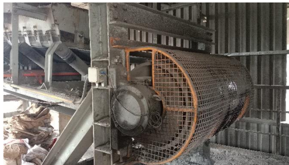
Figure 4. Conveyor belt has installed wire safety as
