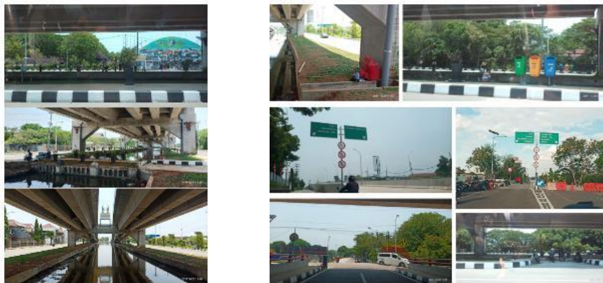
FIGURE 2. Compilation of condition observations at several points in the Madukoro corridor (Source: Author's observations, 2021)
