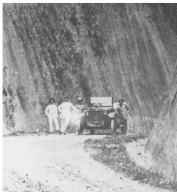
Figure 8. Road of Palembang – Pagaralam Source: ANRI – KIT 511/80 (Arsip Nasional Republik Indonesia, 2009b)
