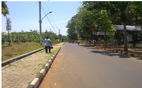
Perkerasan paving block
