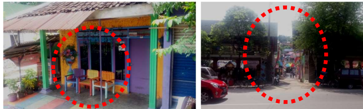
FIGURE 8. Lack of street furniture ( left ) and invisible entrance gate ( right )
