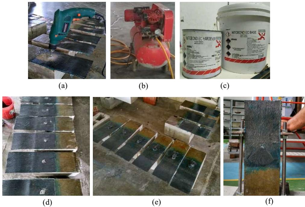
**FIGURE 4.** The installation process of anchored and staked CFRP
