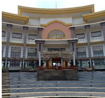
FIGURE 8. A building in Betawi Cultural Village
