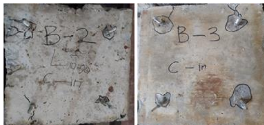
FIGURE 13. Form of Pull-out Failure on Anchor which is close to the edge [2]
