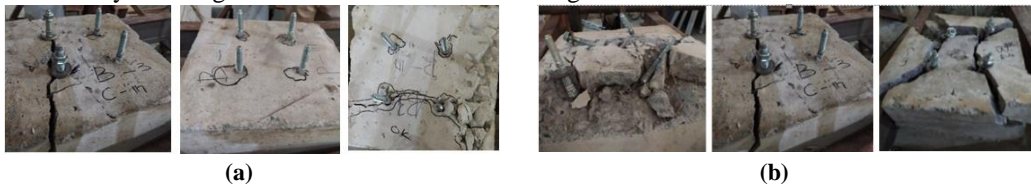
FIGURE 14 (a). Concrete Breakout Damage on Cast in Place Method [5] FIGURE 14 (b). Concrete Breakout Damage on Post Installed Method [5]
