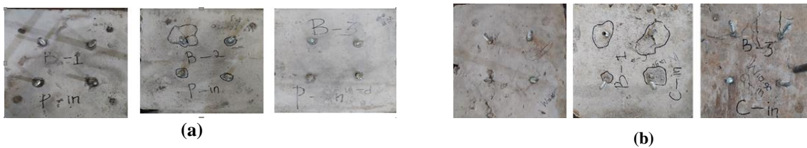
FIGURE 15 (a). Pull-out Failure on Cast in Place Method FIGURE 15 (b). Pull-out Failure on Post Installed Method
