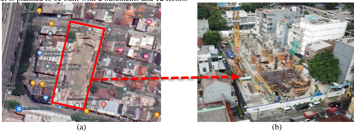
FIGURE 1. (a) The project location is on Kendal Street No.25; (b) Overview of project performance in July 2022
