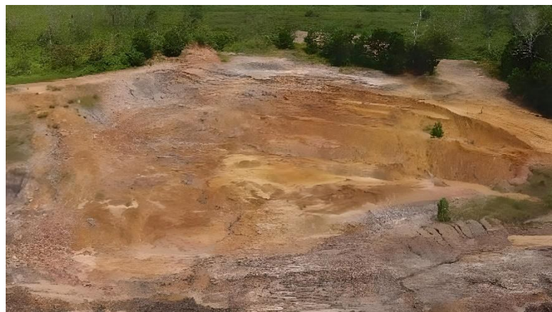
FIGURE 2. Landslide in sections 28+000 to 28+100
