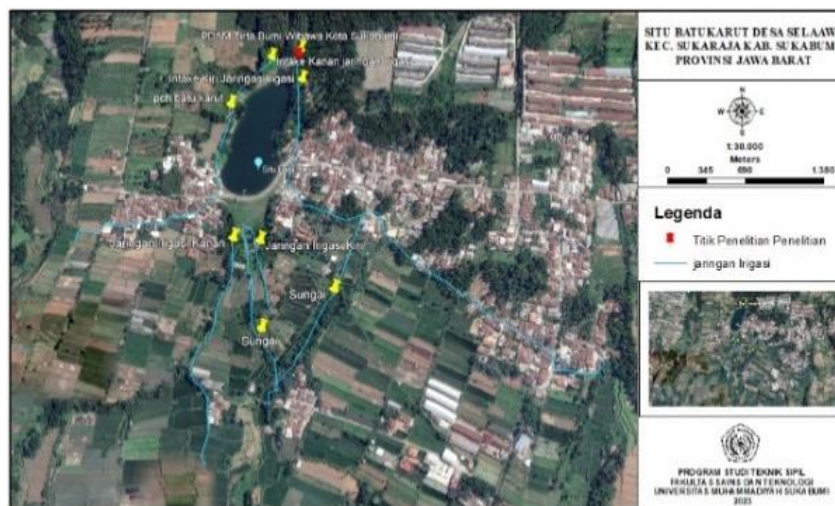
FIGURE 2. Conditions of the study location.
