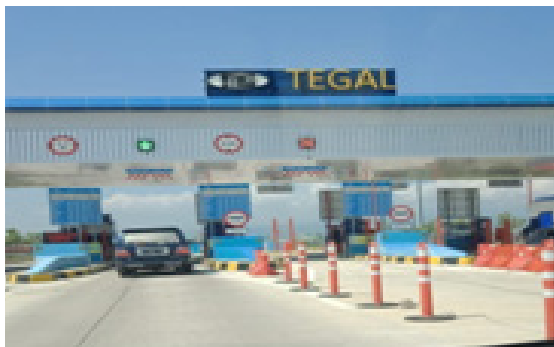
Figure 1. Pejagan-Pemalang Toll Road in Kalimati Village Area (Source : Documentation of Research, April 6th 2019)
