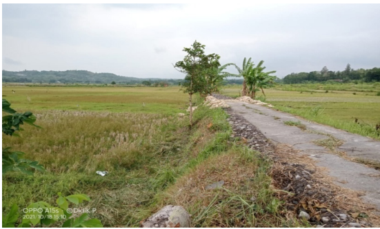
Figure 4. Road conditions before road talud work
