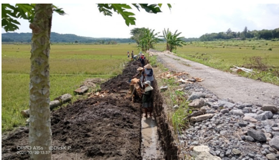
Figure 5. Development conditions 40% of the construction of talud farm business roads
