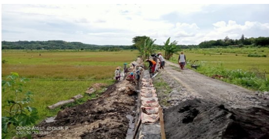
Figure 6. Talud construction reaches 80%
