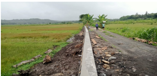
Figure 7. The construction conditions of the talud reach 100%
