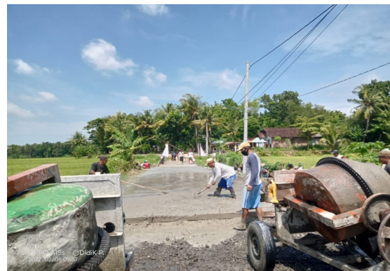
Figure 2. The construction process of the corblok road with PKTD Donotirto Hamlet RT 1
