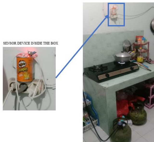
Figure 10. Simulation of the installation of sensor devices in the kitchen
