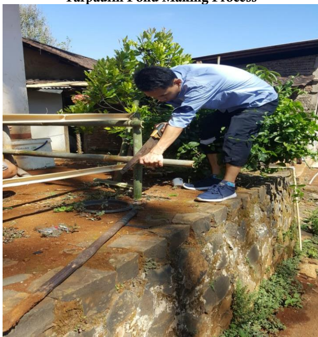
Figure 1. Tarpaulin Pond Making Process
