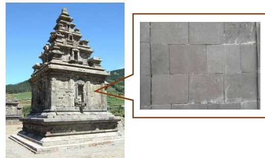
Figure 2. The Connection of Rectangular Material to the Wall of Arjuna Temple
