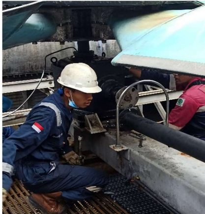
Gambar 6. Melepas Cooling Tower Axial Fan (2)
