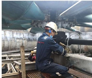
Gambar 5. Melepas Cooling Tower Axial Fan
