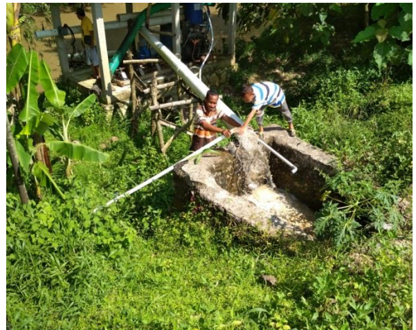
Gambar 5. Debet Air Mobile Pompa Tenaga Surya
